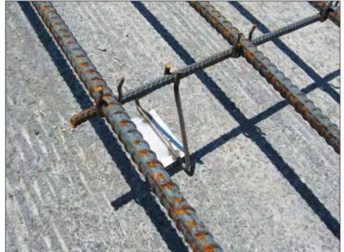
Figure 34. Transverse bar assembly (TBA).
