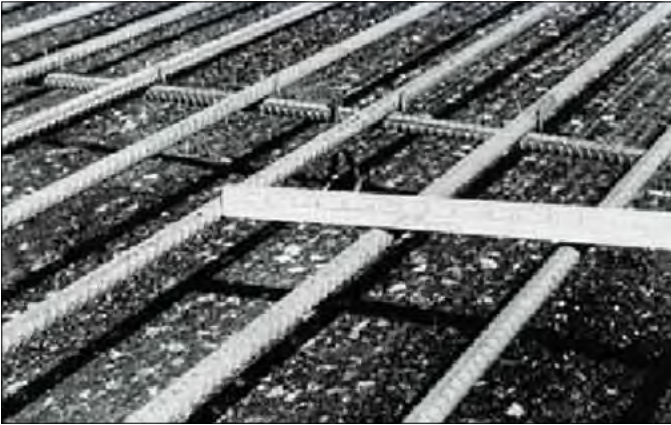
Figure 60. Lateral spacing of longitudinal steel.
