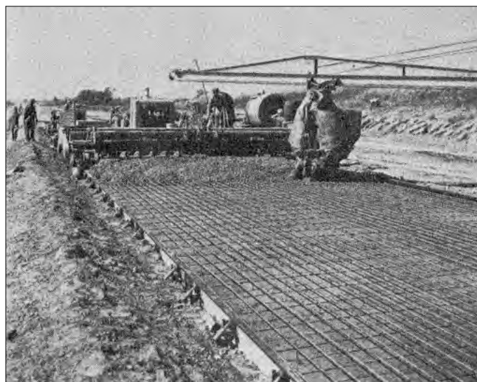
Figure 63. Construction of the 1947 Vandalia CRCP test sections (Illinois).
