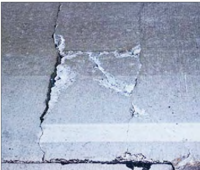
Figure 7. A typical CRCP punchout distress.
