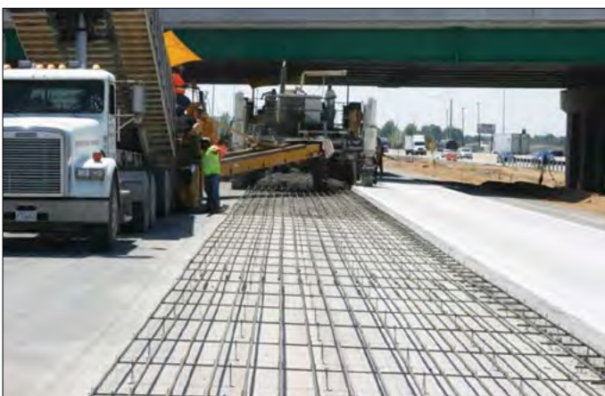
Figure 77. Unbonded CRCP overlay under construction.
