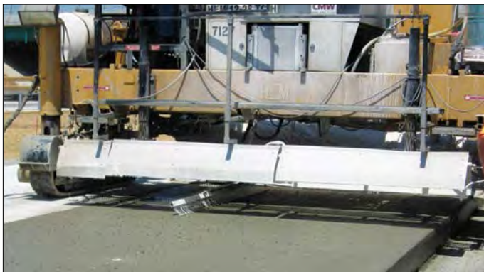
Figure 39. Applying transverse tining on a new CRCP.
