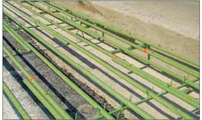
Figure 28. Longitudinal construction joint with tie bars.
