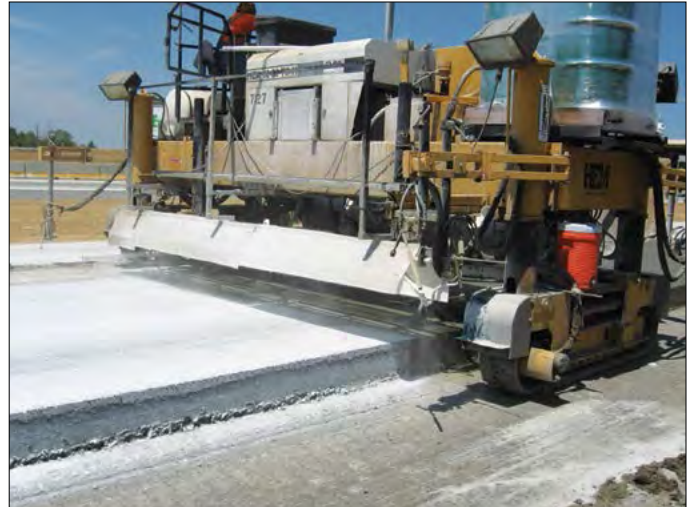
Figure 38. Application of curing compound on slip-formed CRCP.
