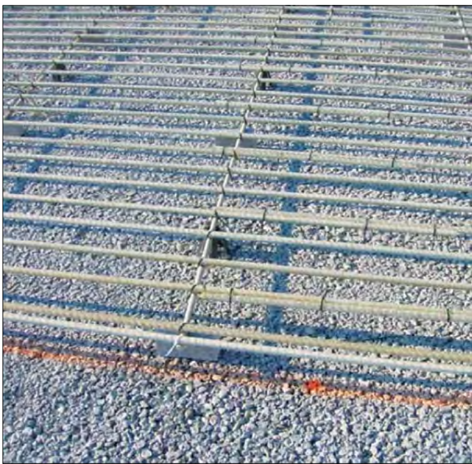
Figure 65. GFRP longitudinal reinforcement for CRCP (Canada).
