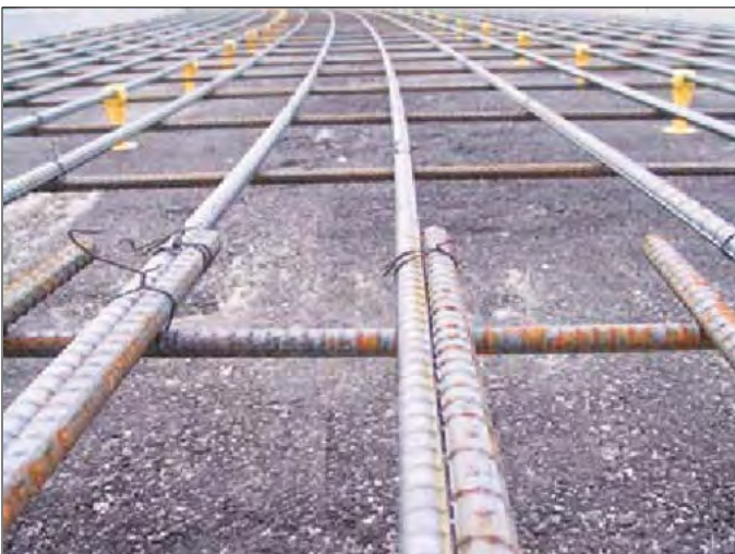
Figure 24. Lap splices.
