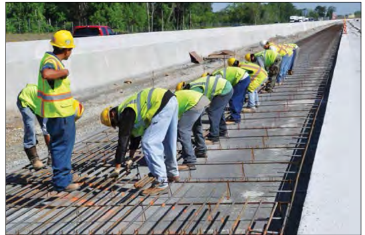
Figure 35. Placing longitudinal steel on TBAs.
