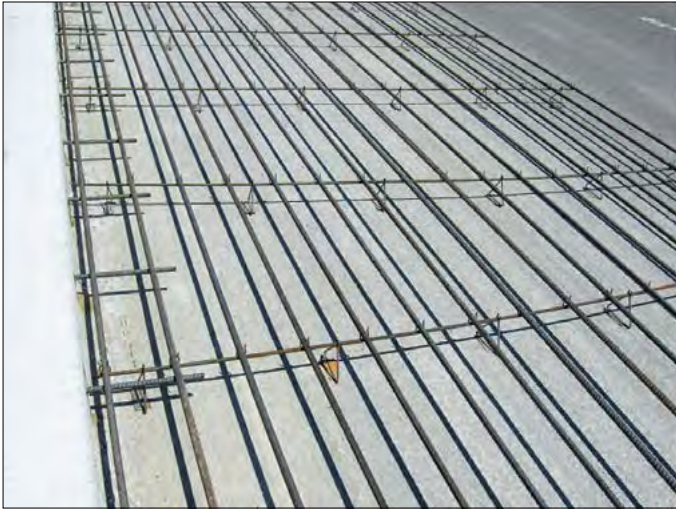
Figure 33. Steel placed on transverse bars assemblies (Illinois).
