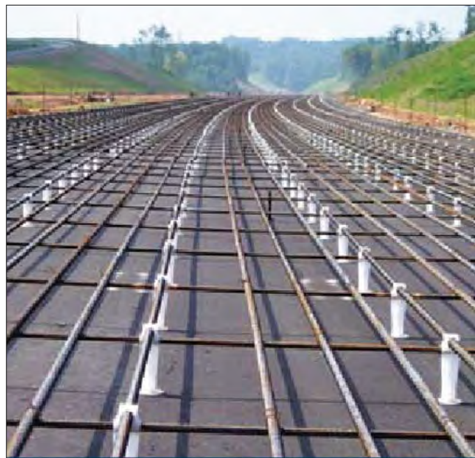
Figure 22. Steel placed on ATB (Virginia).
