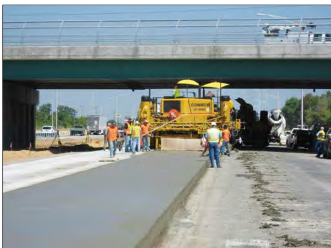
Figure 36. Slip-form paving of CRCP (Illinois).
