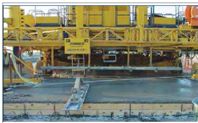
Figure 45. Finishing concrete at end-of-day header.
